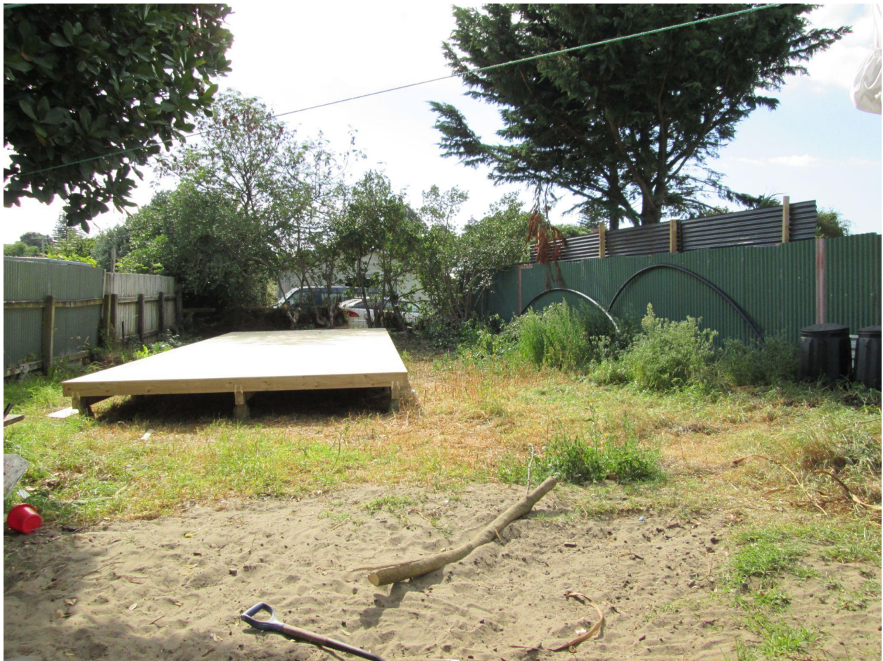
The completed platform before the building's arrival.
