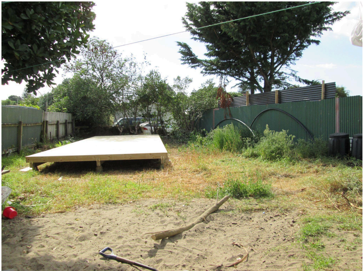
The completed platform before the building's arrival.
